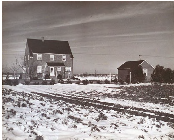
The Boos home in the early 1940s, prior to the construction of Levittown. Levitt & Sons purchased 4,000 acres of potato farms from the Town of Hempstead in 1946, which would later be used to build 17,447 Levitt homes between 1947–51. The land was relatively cheap because the potato fields had been affected by the Golden Nematode, an insect from Europe that destroyed much of the crops at the time. (Credit: Howard Boos)
