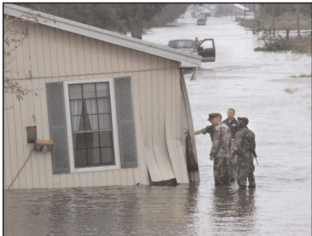
Hurricane Katrina flooding.
